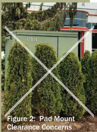
Figure 1: Clearances to Pad Mounted Equipment
